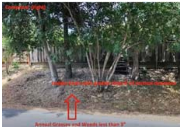
Compliant roadside conditions
